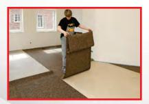
Move to the opposite side and carry out the same process. Once the first strip is complete, move onto the next, adjacent strip ensuring and checking that each strip is tightly butt-joined with no overlaps and NO GAPS.
